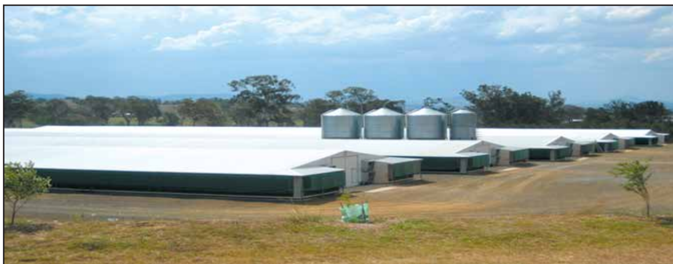
Poultry farm by EPS Sandwich panel Shed
