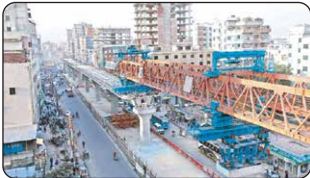
False Work Support of Metro Rail, Mirpur, Dhaka
