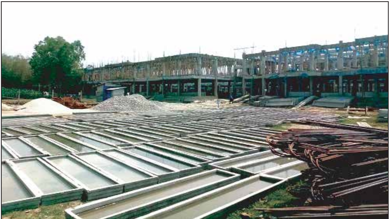
Ferrocement Slab casting for Roof Work
