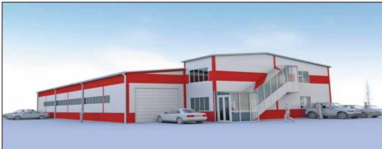
Air Conditioned Factory Shed by EPS Sandwich Panel
